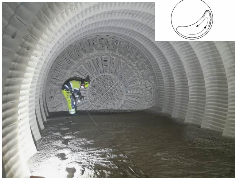
b) Cascading of grinding media (Chamber 2)
