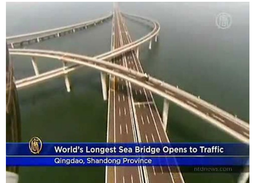
Jiaozhou bay bridge - 40 km
